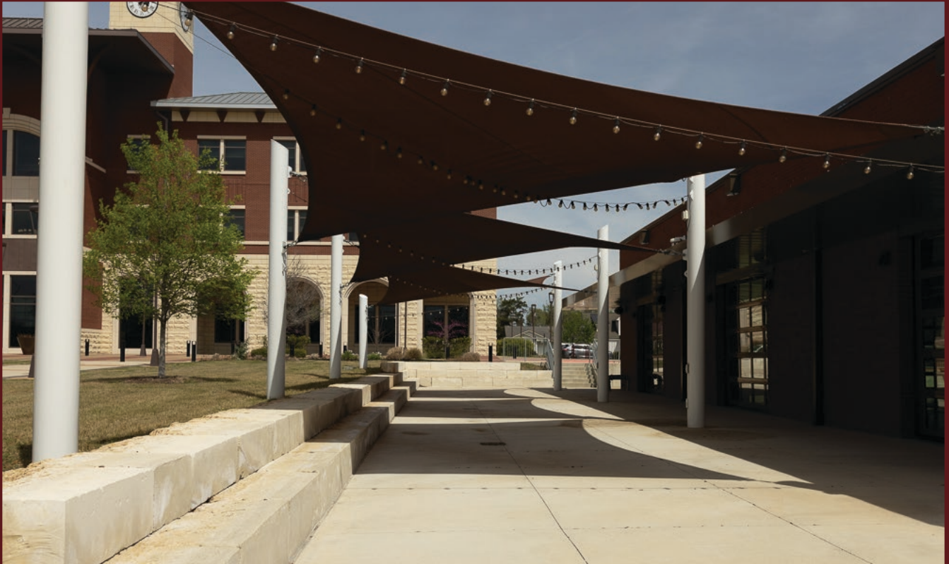
Figure 4.16 City Hall Structured Shading
